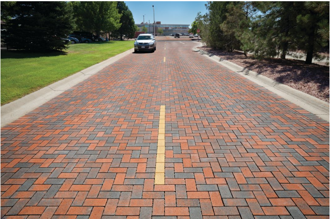
| Thule Street contains 18,000 square feet of pavers.
